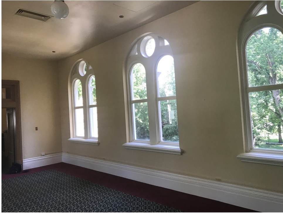
Breezeway – north wall
